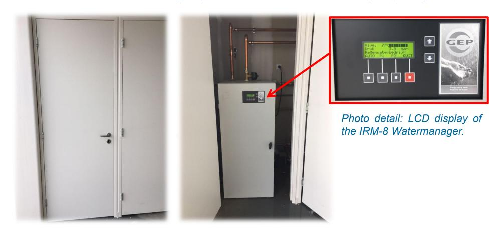
The IRM-8 Watermanager is equipped with a automatic control system with LCD-display which controls the system as well as the automatic cleaning of the rainwater filter.
