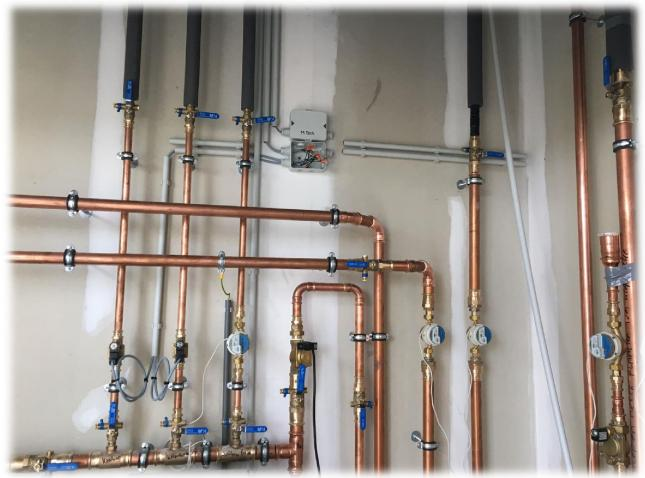
Nice piece of quality installation. Water gauges are placed to monitor the water flows, magnetic valve is placed for the automatic filter cleaning.
