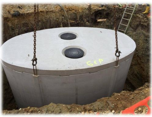
The Varitank Flexoline rainwater tank is made of concrete and has a total volume of 20.000 liters. The bottom part is completely made out of a single piece. Tank is equipped with 4 lifting rings and 2 prefab installed man-holes. The filtershaft has a filter capacity of 1.650 m2 of roof surface. The filter grid is made with the special Trident technology.
