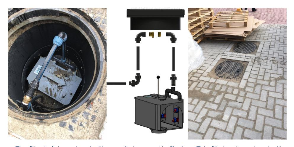
The filtershaft is equipped with a vertical removable filterbox. This filterbox is equipped with automatic filter-cleaning which cleans the filtergrid periodically. Child-safe covers are placed on . the manholes.
