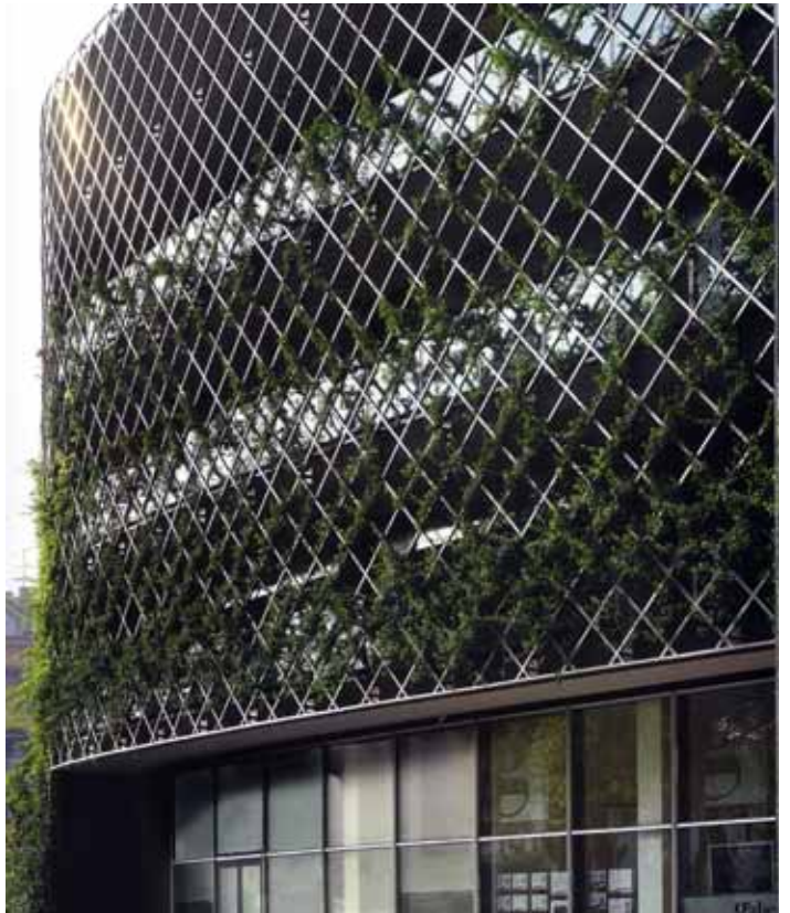
Ex-Ducati Building, Rimini, Italy (Photos sourced from Lambertini & Leenhardt)
