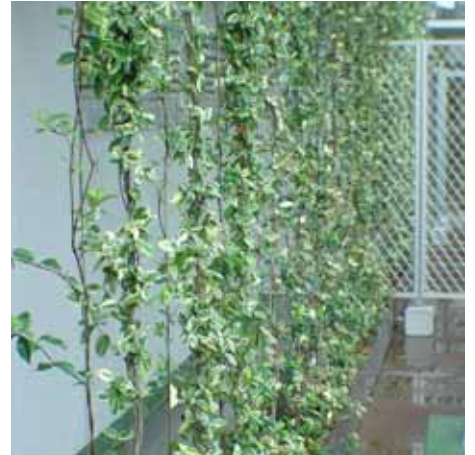
Cable system with climbers in Japan (Photo sourced from Fifth Creek Studio)
