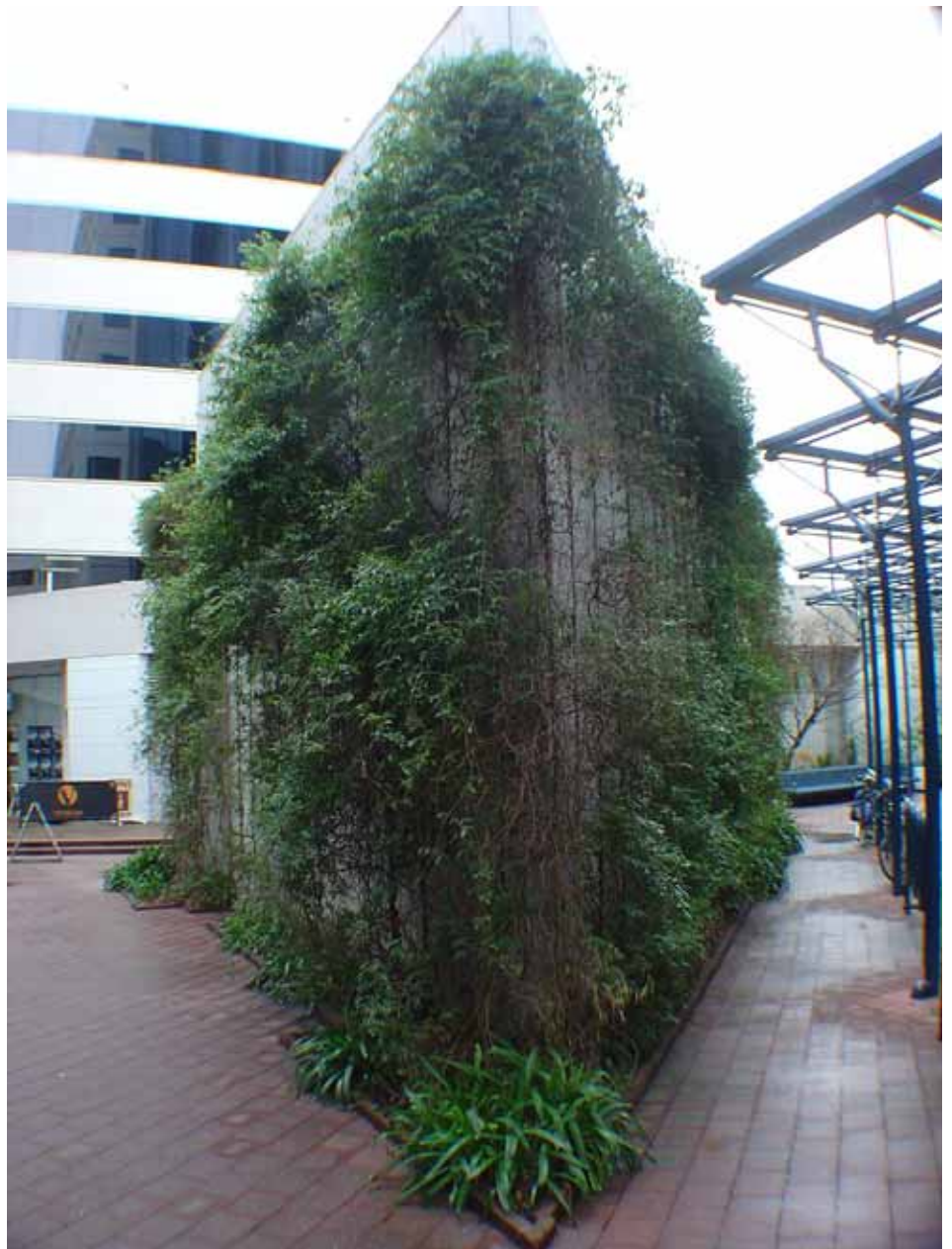
Capital Centre, Canberra living wall after 25 years - designed and constructed by Graeme Hopkins (Photo sourced from Fifth Creek Studio)
