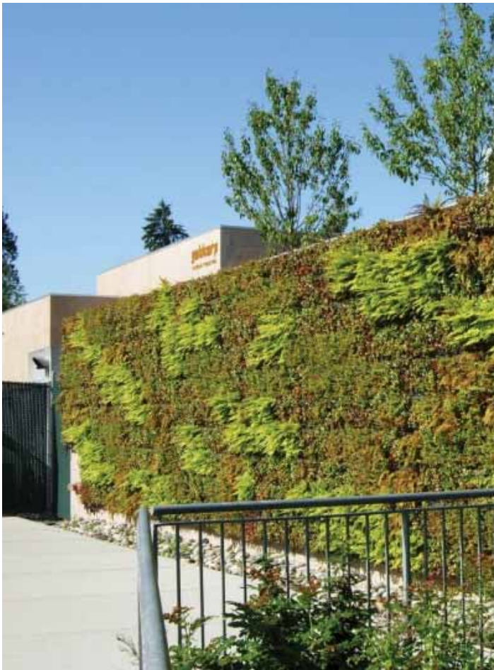
Vancouver Aquarium (Photo sourced from Living Architecture Monitor)
