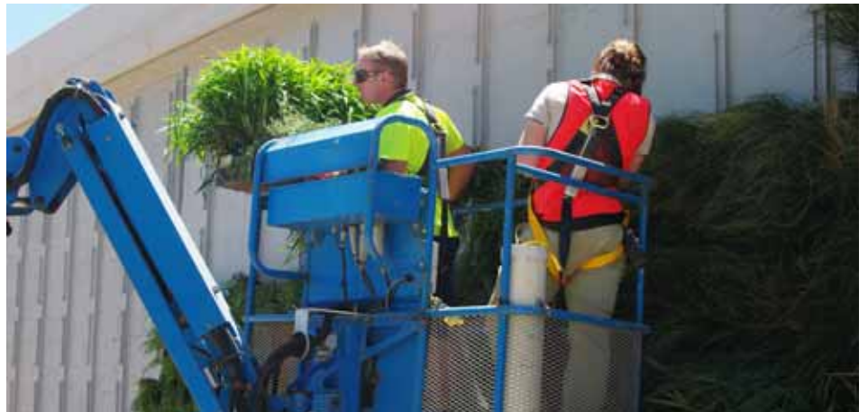
Adelaide Zoo living wall installation using a forklift system (Photo sourced from Fifth Creek Studio)
