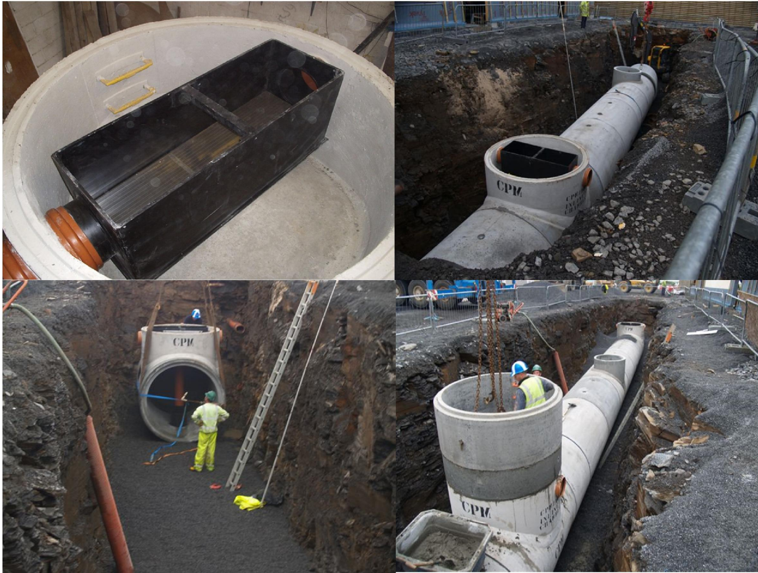
Trident 6000 Regenwaterfilter in 60.000 L tank.
